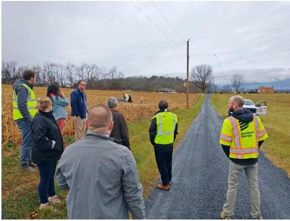
Jimmy Carr of APB and Dominion Energy representatives describe the process of last-mile cable installation and pole replacement. The private road has several homes that will be served by this fiber cable feed.
