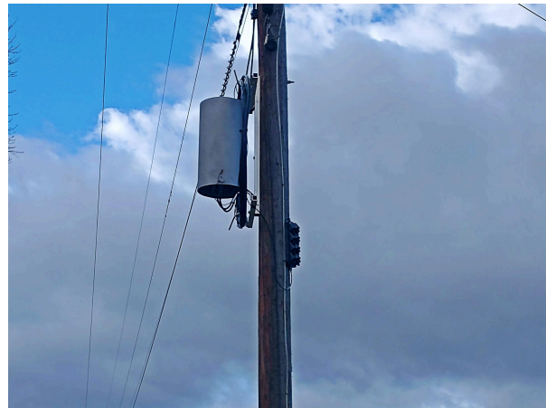
These gray cross-connect canisters will be installed on poles throughout the system to connect the distribution cables.
